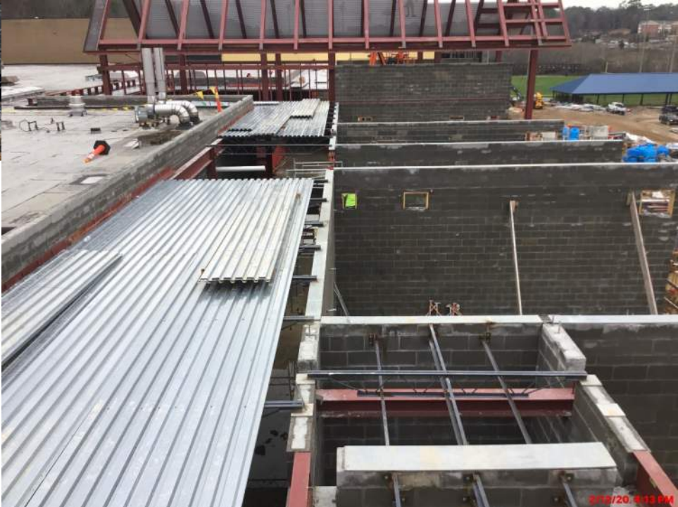
Classrooms – Joists & Decking
